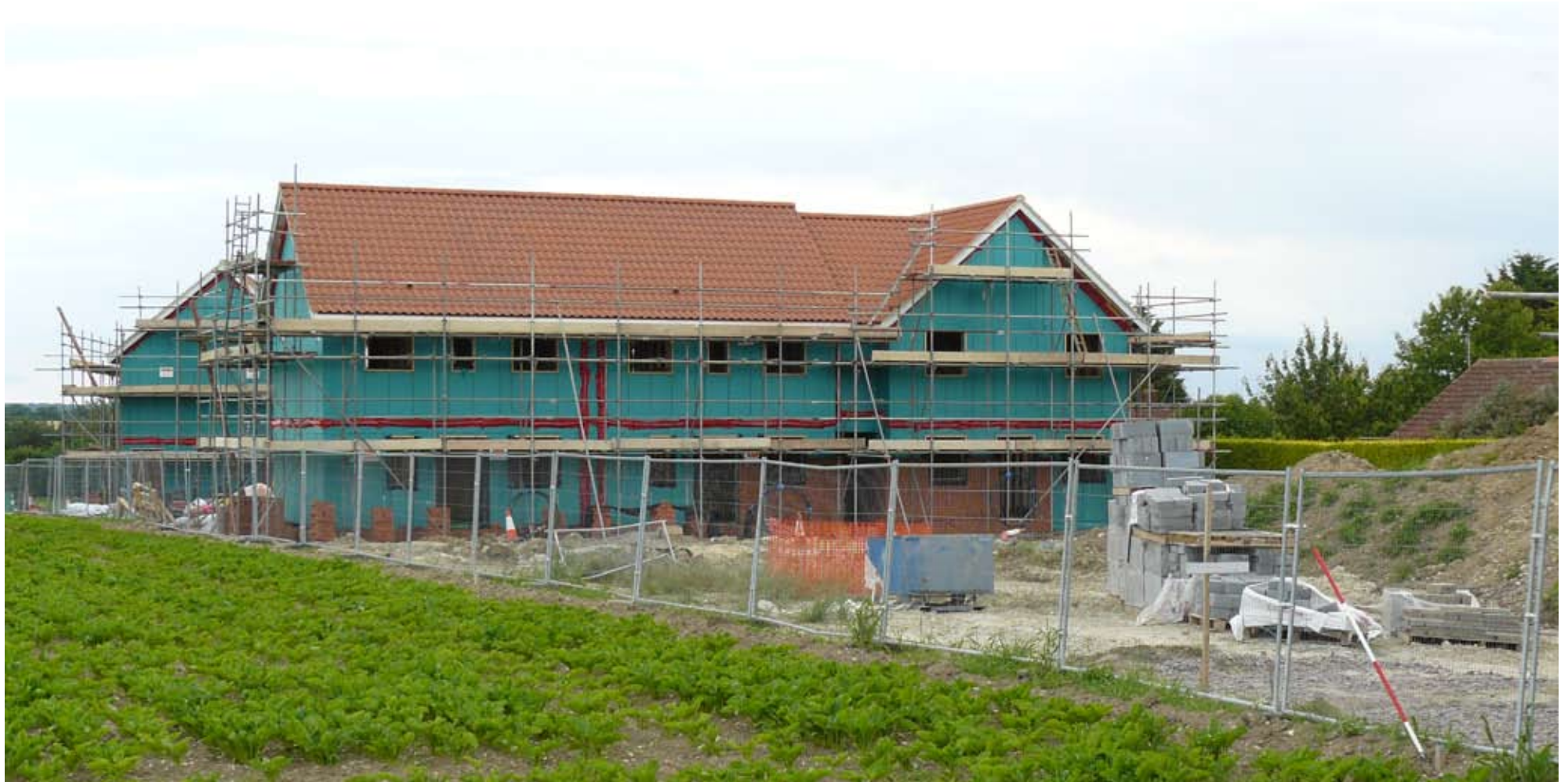
New social housing at Langham under construction
