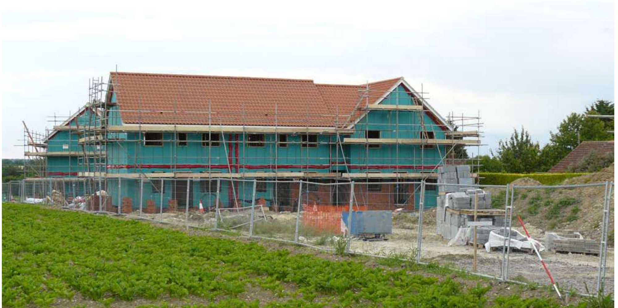
New social housing at Langham under construction
